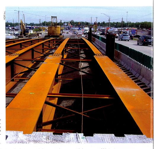
Allowing the contractor to install the shear studs in the field rather than having them installed in the shop as is traditionally done with cast-in-place decks provided greater tolerance for the erection of the deck panels and facilitated their placement.
