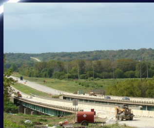
Boone County Overlay 700' x 30' Twins Brad's crew overlayed these twin bridges.
