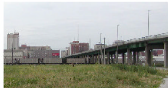
HARRIS OVERPASS, LINCOLN, NE REPLACE 1900' VIADUCT CONTRACT: $18,000,000 START: 11-12-07
