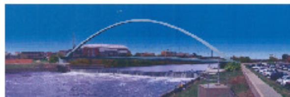
CENTER ST ARCH PED BRIDGE, DSM, IA NEW 400' STEEL ARCH CONTRACT: $9,500,000 START: 8-15-07
