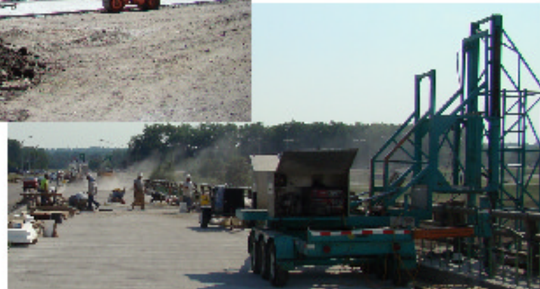
2311' US 63 River Bridge Ottumwa
