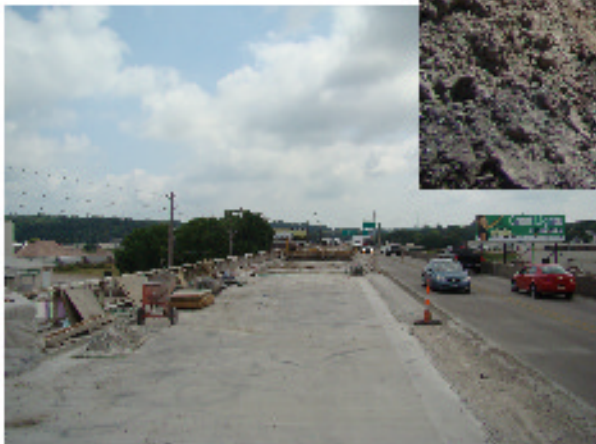
3970' Gordan St Viaduct Sioux City
